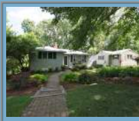
4015 Lawrence Ave, Kensington/Rock Creek Palisades Sold - August 30, 2011 $290,000
