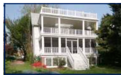
10405 Fawcett St., Kensington Historic Kensington $925,000
